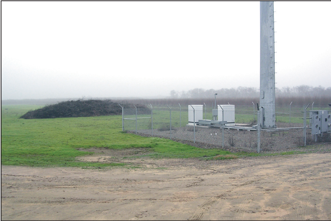
Photo 5, Site W-2 View from southeast corner of parcel looking west.
